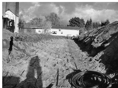
Figure 5.30 Installation of ground heat exchangers
