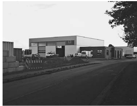
Figure 17.6 The hall with adjacent offices
