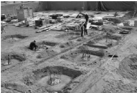
Figure 5.18 Energy posts installed as foundations
