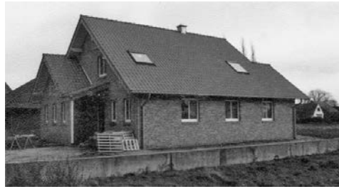
Figure 17.8 Commissioning a heat pump in a detached family house
