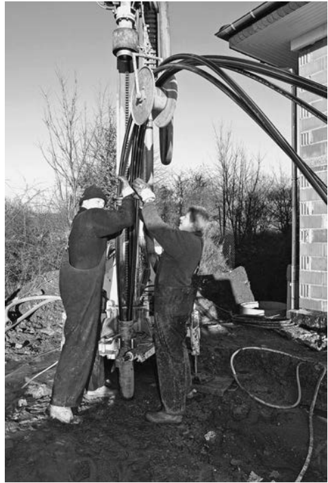
Figure 5.17 Installing borehole heat exchangers
