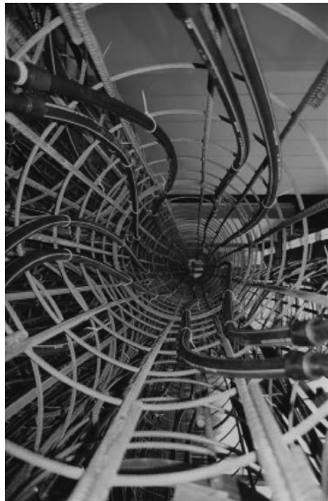
Figure 5.19 Energy post prior to installation
