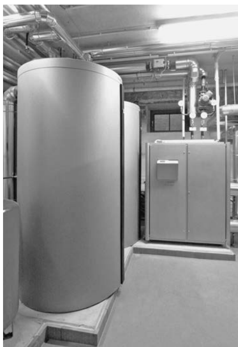
Figure 17.2 Example of two-stage heat pump system for high flow temperatures, manufactured by Viessmann
