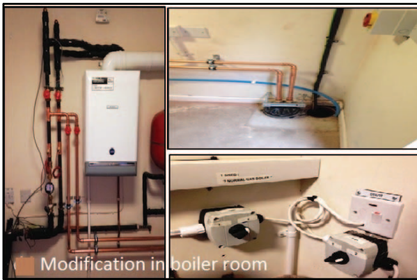
Fig. 5 Modification in boiler room with existing system
